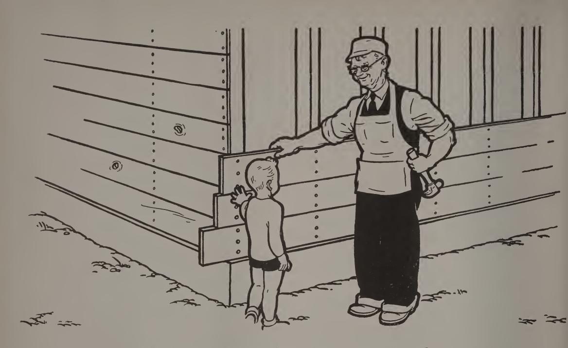
When all the uprights had been put in place and the frame of the house was completed, long boards were nailed on the outside. Each board was nailed to the uprights. If the boards were too long, they were sawed off after they had been nailed in place.
